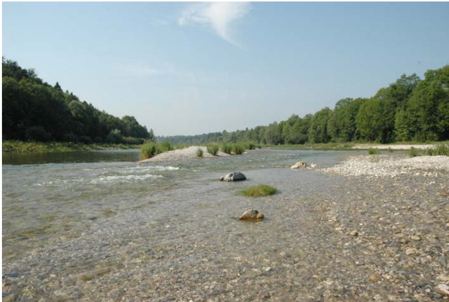
Fig. 3: Broadening of the main channel bed
